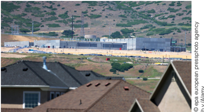
FIGURE 2.17 The NSA data center in Bluffdale, UT.
