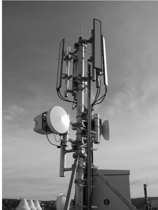
Figure 13-4: A Base Station Sector Antenna Array (Courtesy of European Antennas Ltd.)
