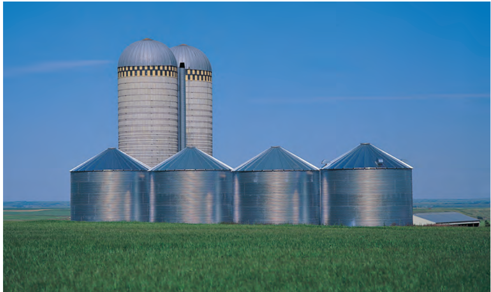
Figure 2.7 Grain silos – a great analogy for the problems of separate applications and databases
