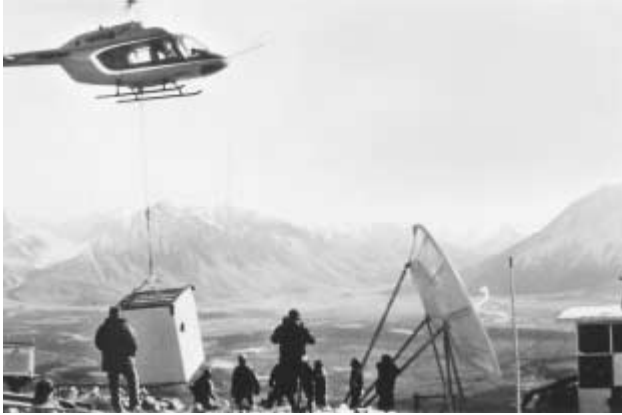
Figure 14.7 Transportable message station. (From Telesat Canada, 1983. )
