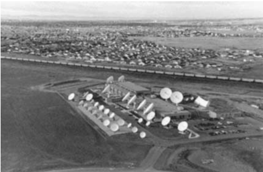
Figure 16.9 Uplink facilities for Echostar's DISH network. (From http://www.dishnetwork.com/profile/third level content/uplink center/index.asp .)
